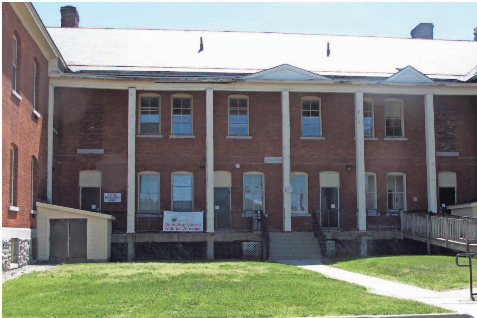
The entrance to the Dupont Building from parking on Hegeman Avenue in Colchester.
